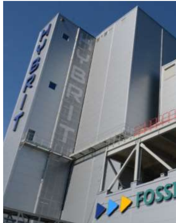
World-unique pilot plant started operation in 2020.
